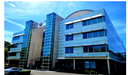
BMW Group Headquarters in Farnborough
